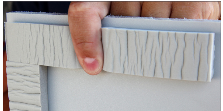
Each door has 1” wide weather stripping attached to the back to insure a tight air seal between the door and the home.
