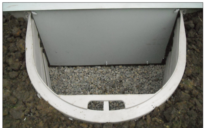
An access well can be installed, if any part of the door is below grade.
